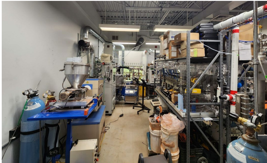
Figure 1: Pilot plant setup at the Boucherville facility
