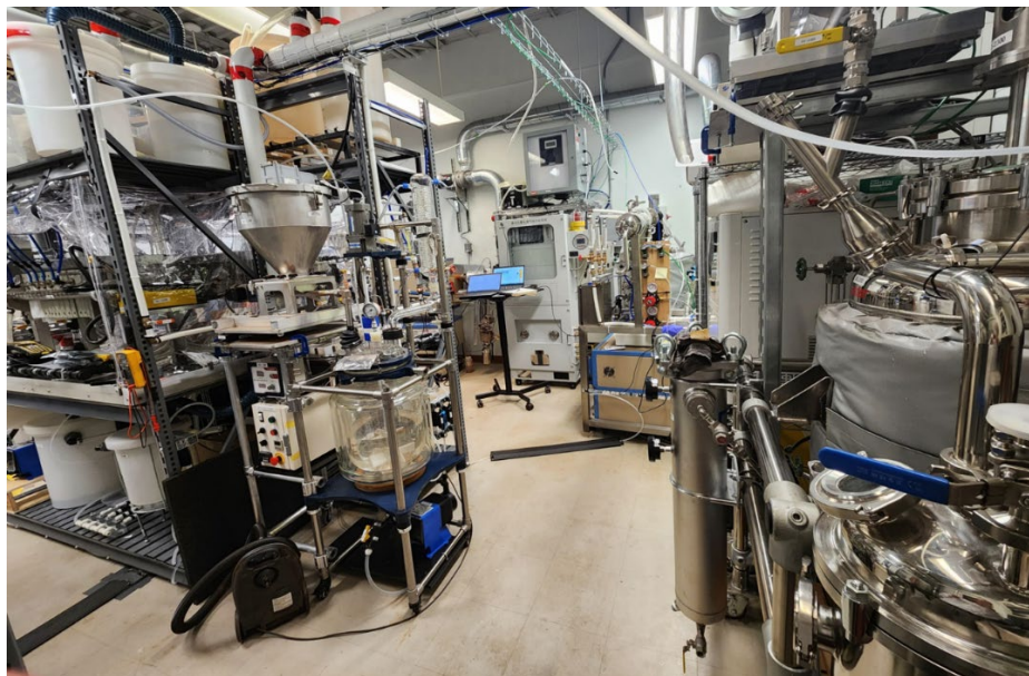
Figure 2: Pilot plant setup at the Boucherville facility
